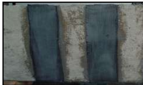
8.29-rasm. To'sin o'ralgan polosaning oxirgi bosqichi
