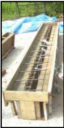
8.20-rasm. Tavr shaklli to'sinni yog'och qolipda tayyorlash
