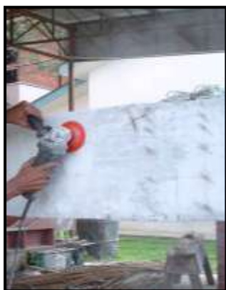
8.25-rasm. Betonli to'sin yuzasini mexanik maydalagich yordamida tayyorlash
