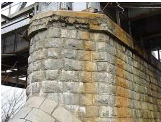
5.50-rasm. Ko‘prik oraliq tayanchi fermaosti plitasi armaturasining yalang‘ochlanishi bilan beton singan bo‘lagi
