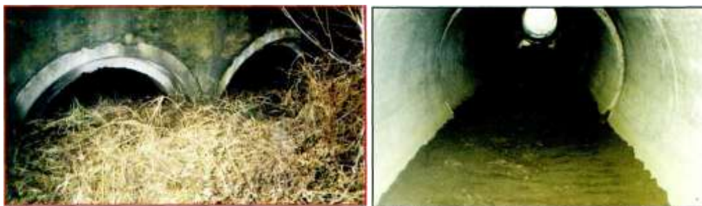
5.16-rasm. Suv o'tkazuvchi quvurning loyqa bosishi
