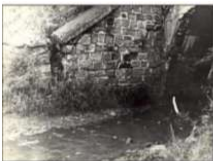
5.10-rasm. Quvur kallaklarining qisman sinishi: a – tirgak devorining; b – qanotlarining
