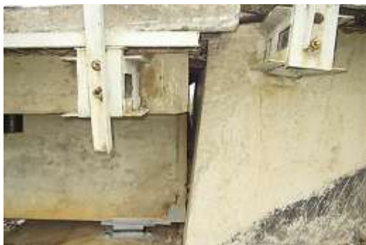
5.52-rasm. Ko'prik qirg'oq tayanchining qiyshayishi
