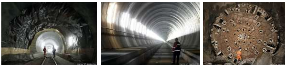
Tunnelning ko‘rinishi va ulkan Sissi burg‘ilovchi ustanovka
