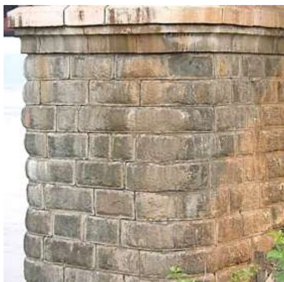
5.49-rasm. Tayanch qoplamasi choklarining emirilishi
