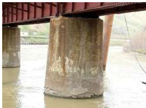
5.53-rasm. Ko'prik oraliq tayanchining qiyshayishi
