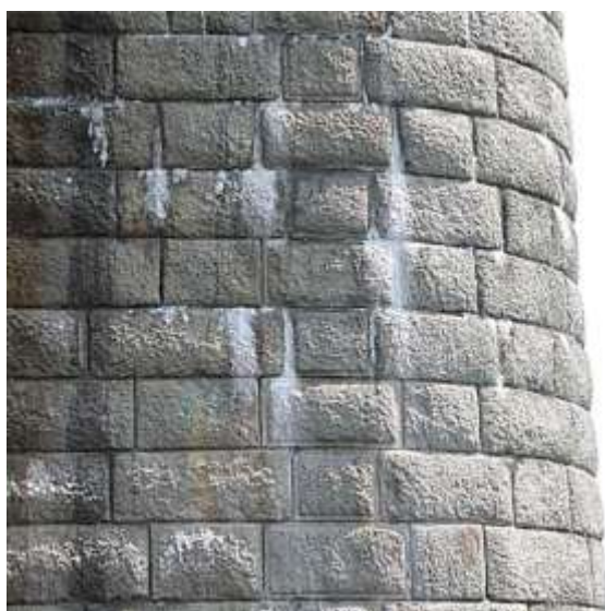
5.48-rasm. Tayanch qoplamasining choklari bo'yicha ishqorlanishi
