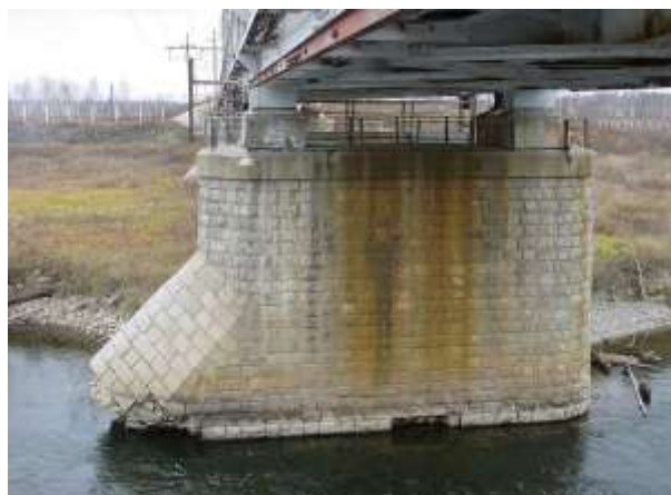
5.51-rasm. Tayanchning yuvilishi natijasida sinishi
